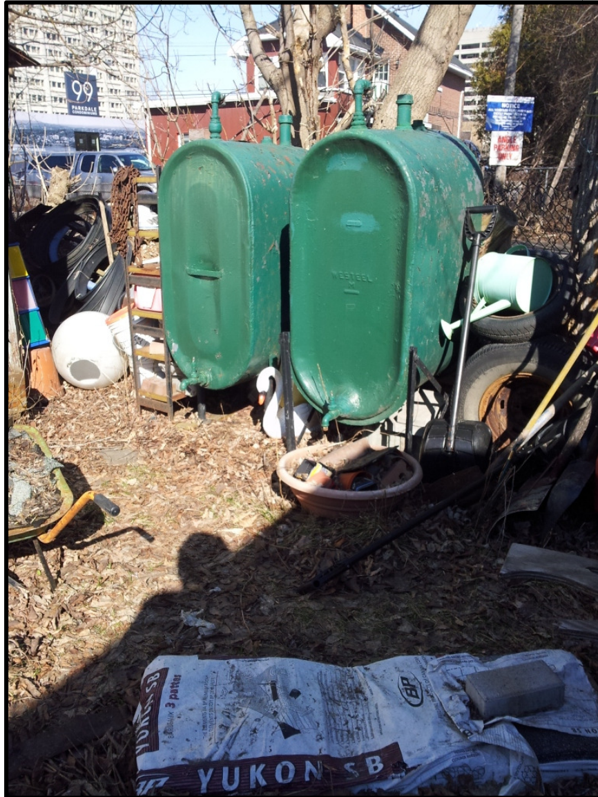
Photograph 1: ASTs on the exterior of the subject site (266 Parkdale).
