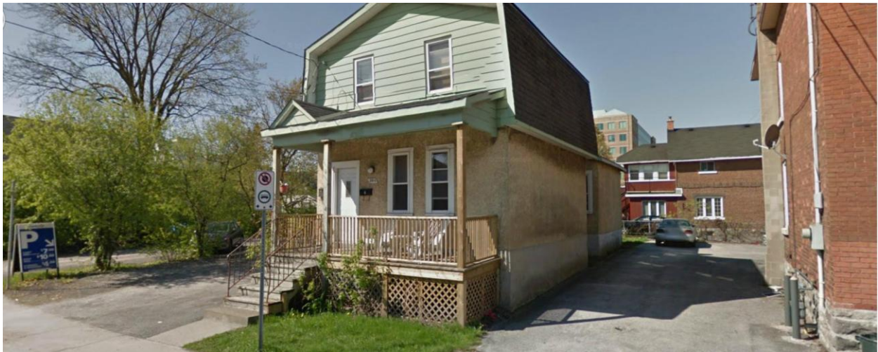
Figure 8: Looking west at 254 Parkdale Avenue
