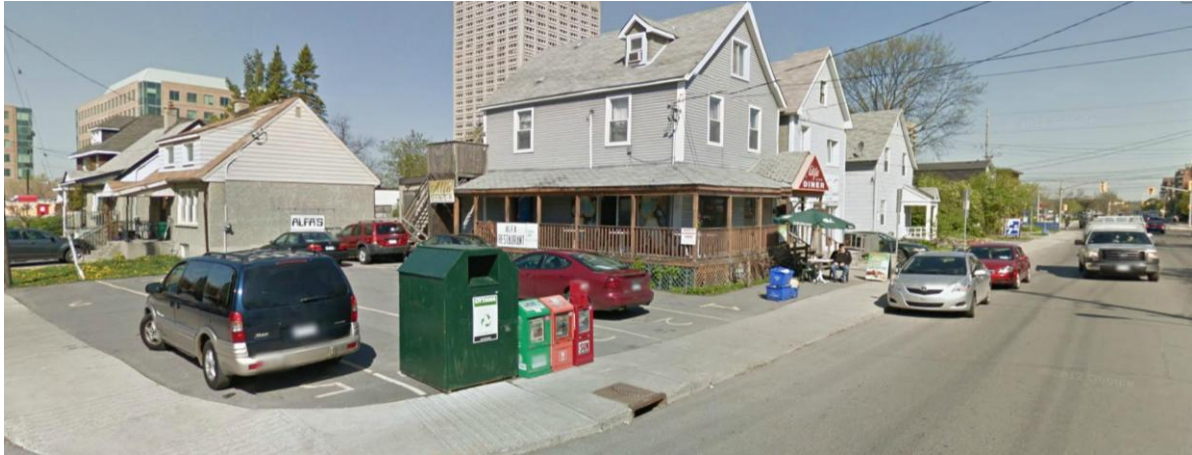
Figure 10: Looking northwest from Parkdale Avenue and Bullman Street
