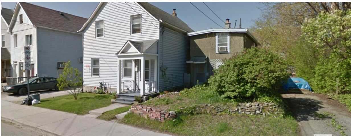
Figure 9: Looking west at 268 Parkdale Avenue
