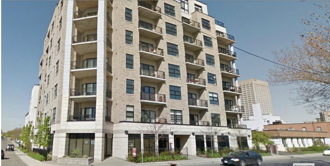
Figure 14: Mid-rise development (7 storeys) at 45 Spencer Street
