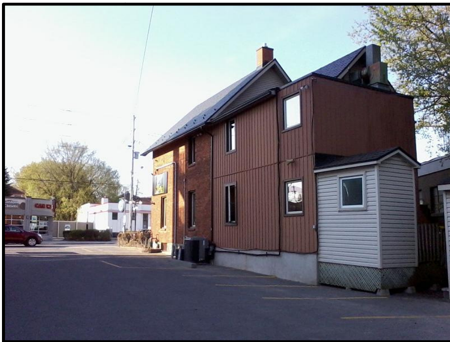
Photograph 10: Building at 1445 Wellington Street West, facing southwest.
