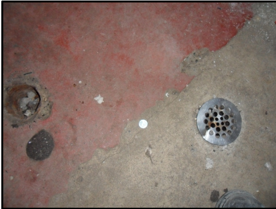
Photograph 7: View of the furnace room floor. Photograph illustrates 200 mm floor drains.
