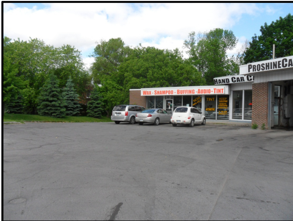
Photograph 2: View of remainder of the subject structure's south side, looking northwest. Photograph illustrates the building addition (1975), and vacant grassed/treed land to the west.
