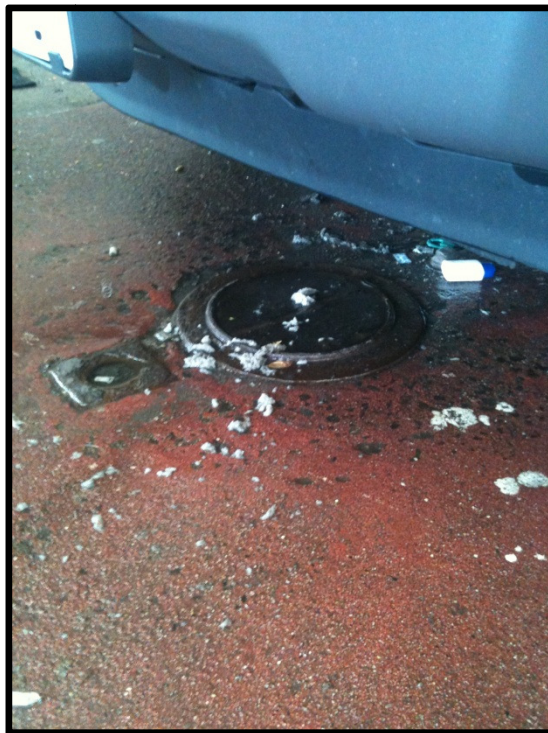
Photograph 8: View of floor of former garage bay. Photograph illustrates former in-ground hoist.
