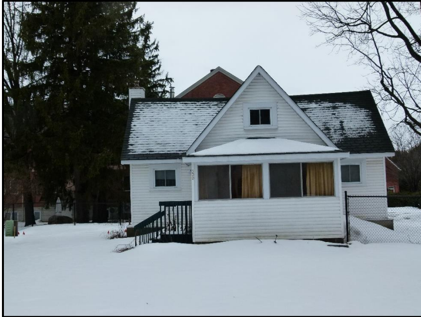
Photograph 1: 530 Edison Avenue (March 28 th , 2017).
