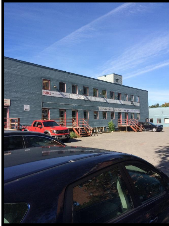
Photograph 1: View of the east building face, looking west.
