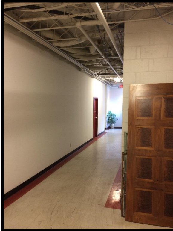
Photograph 5: Typical construction of the building's common hallways.
