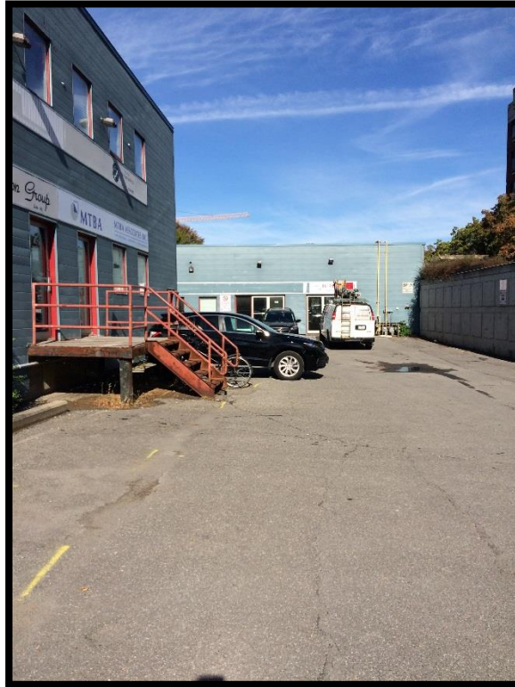
Photograph 3: View of the interior south face of the building, looking north.
