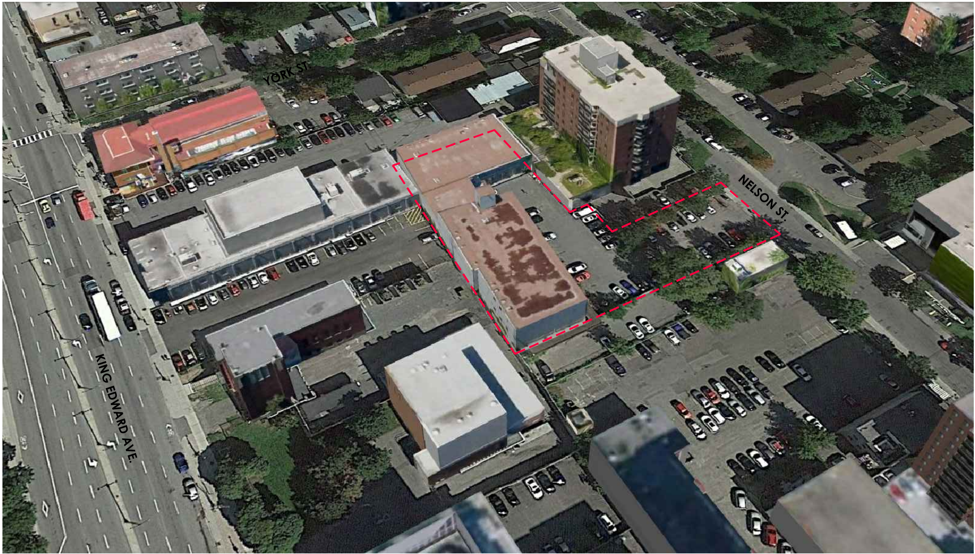
AERIAL VIEW OF SITE LOOKING NORTH
