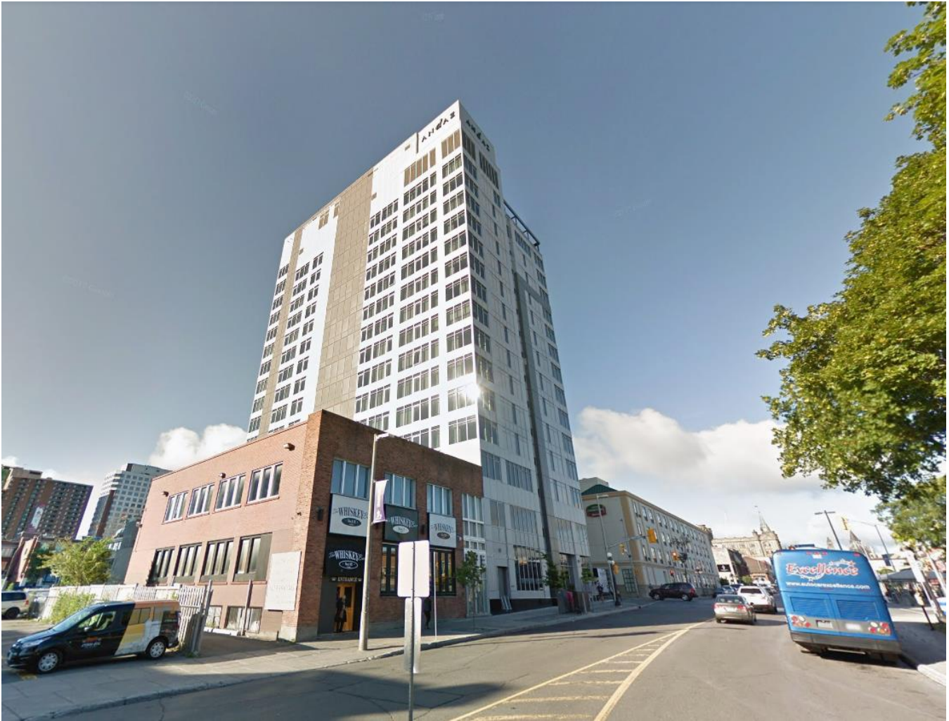
Figure 6: Existing Building On-Site in Context of Present Andaz Hotel
