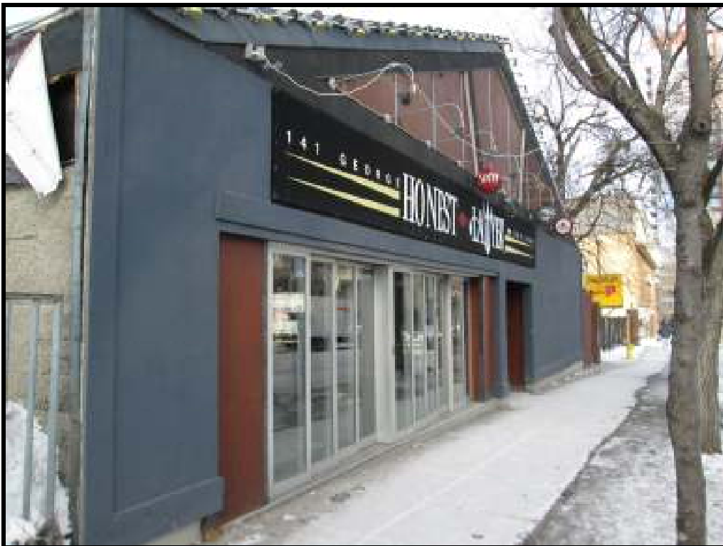
Photograph 6: South wall of structure at 141 George Street, facing northeast.
