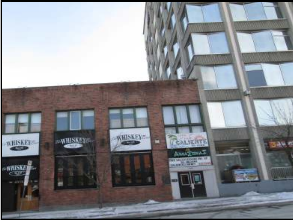
Photograph 3: North wall of 321 to 325 Dalhousie and adjacent property to the east, facing south.
