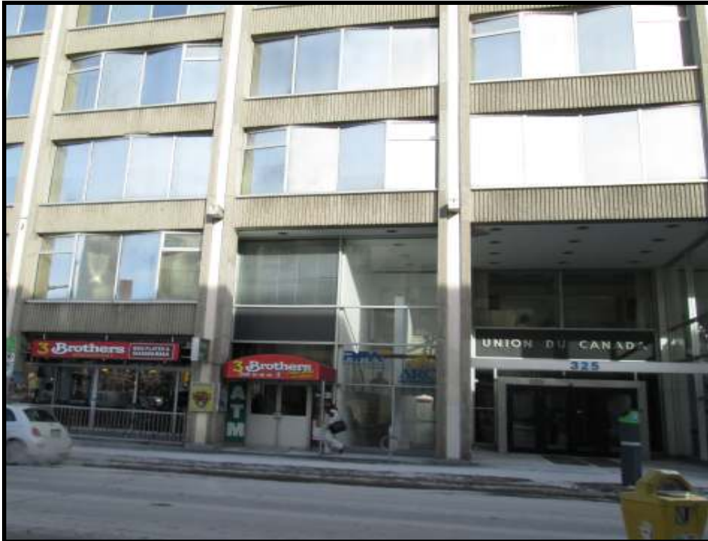
Photograph 1: West wall of 321 to 325 Dalhousie Street, facing east.
