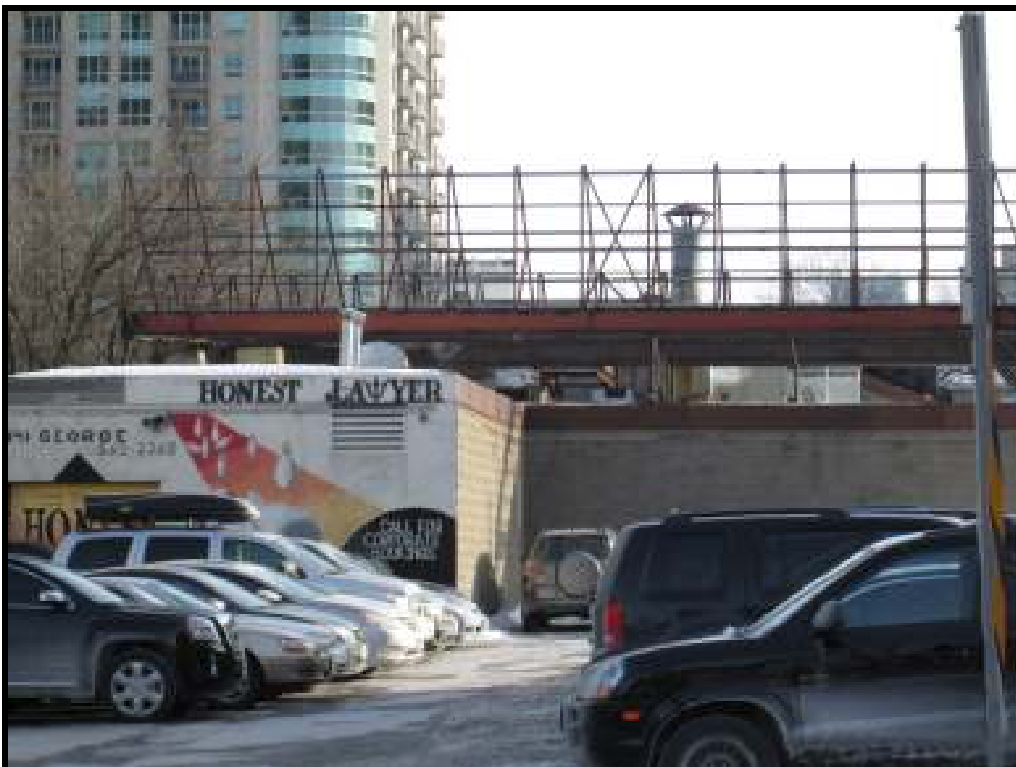
Photograph 8: South wall of structure at 141 George Street and rear addition and parking lot adjacent to the north, facing south.
