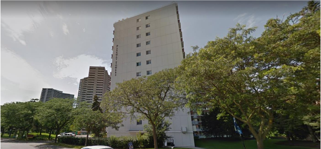
Figure 4: Towers to the West of the subject property.
