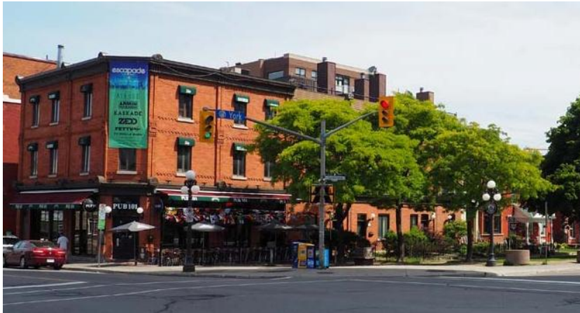
Figure 11: North side of York Street, with 101 York Street on the left (west), built 1898. Photo taken in June 2018. Source: Contentworks.
