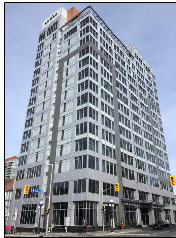
Exhibit D.3 – 325 Dalhousie Street
