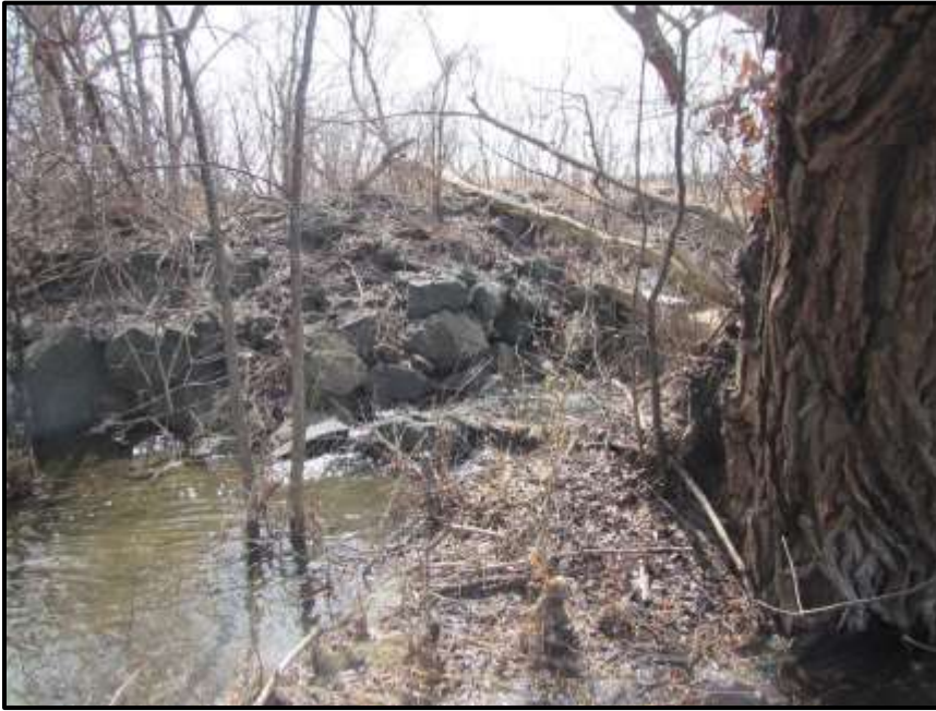
Photograph 7: Old Stone Weir downstream of pond in Survey Site #2 (March 30 th , 2018).
