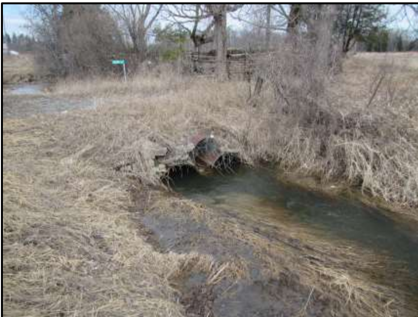
Photograph 2: Survey Site #1 - Three (3) stacked 60 cm CSP culverts under the old farm driveway, east of March Road (facing upstream) (March 30 th , 2018).
