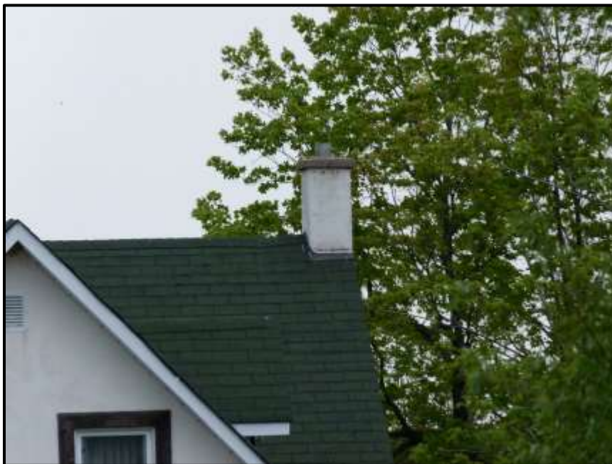
Photograph 32: Chimney at 1035 March Road. Note the metal liner (May 24 th , 2017).
