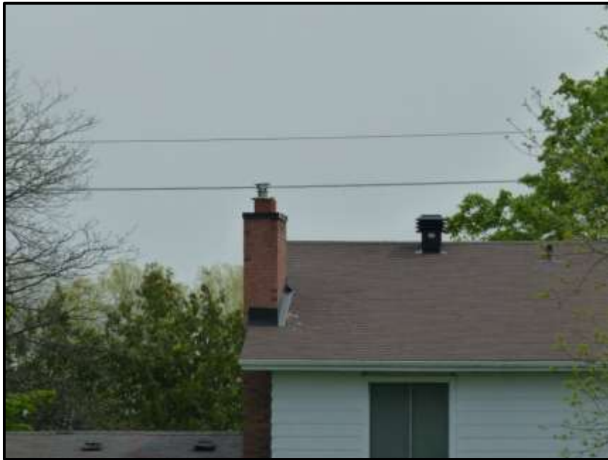
Photograph 33: Chimney at 1053 March Road. Note ceramic liner and metal cap (May 24 th , 2017).
