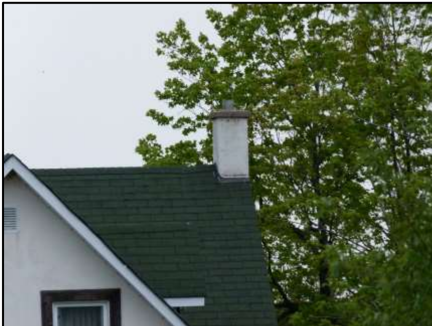
Photograph 32: Chimney at 1035 March Road. Note metal liner (May 24 th , 2017).
