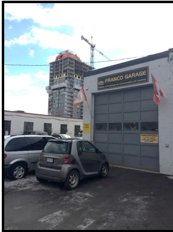
Photograph 1: View of the building front at 70 Beech Street, looking southeast
