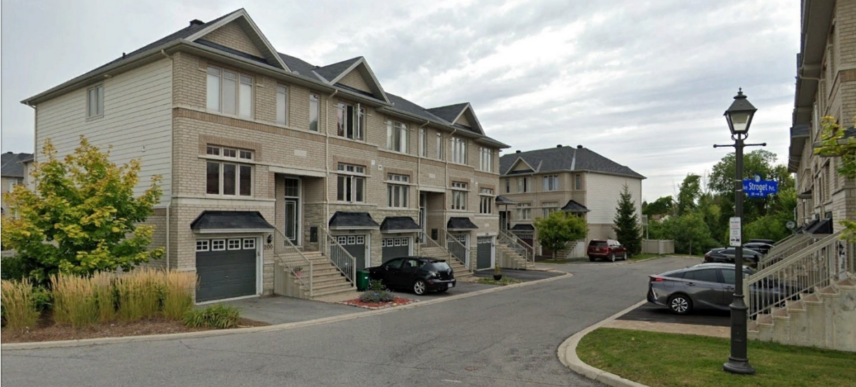
Figure 4.1: Three Storey Narrow Lot Townhouses on Stroget Private, Ottawa
