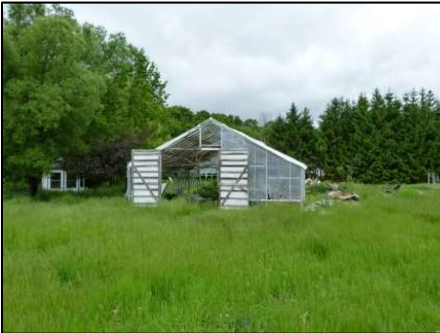
Photograph 7: Looking north at Building #2 (Glass and Metal Greenhouse) (June 11 th , 2019).
