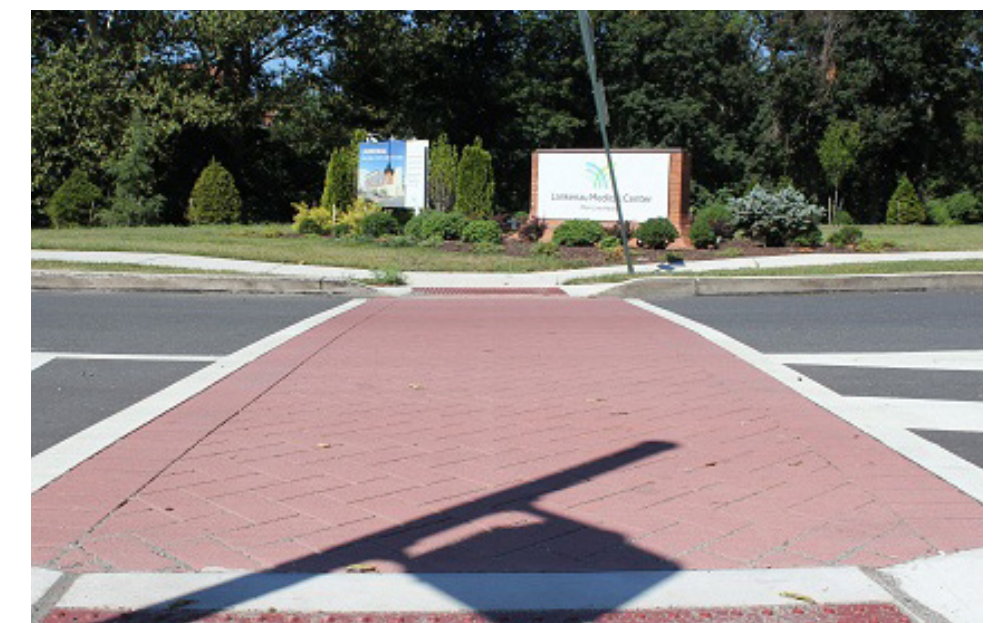
Figure 52 Mid-Block Pedestrian Crossing Example
