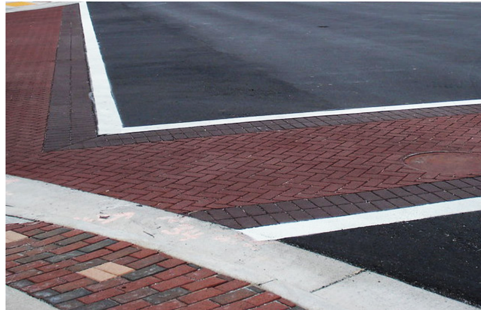
Enhanced Intersection Paving
