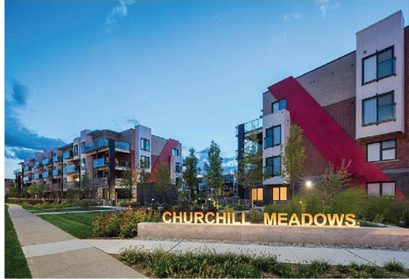
Gateway Entry Feature
