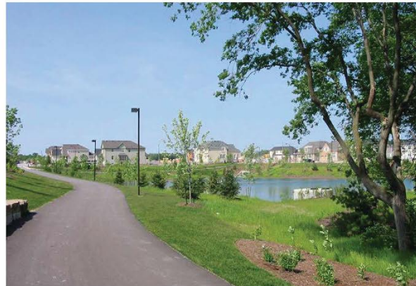
■ Backing Storm Pond Condition
