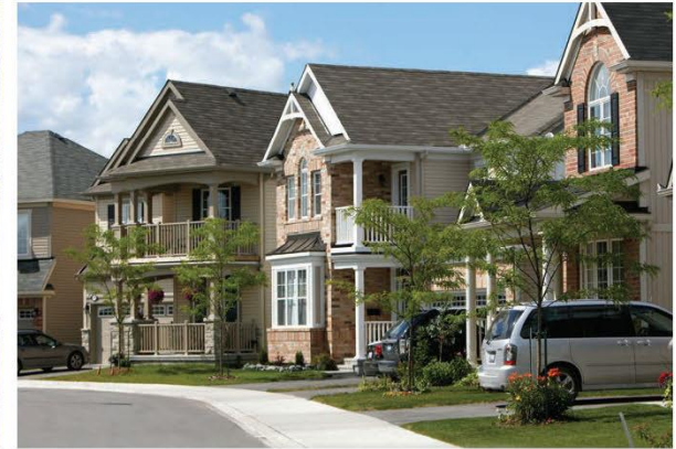
Primary Sidewalk Condition
