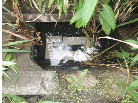
Figure 2b: Water level logger installation at Q2
