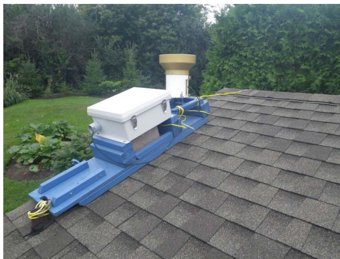
Figure 2e: Rain gauge installation
