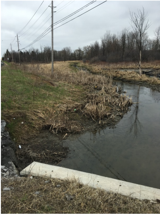
13. KDG-1 looking downstream from Carling Avenue.
