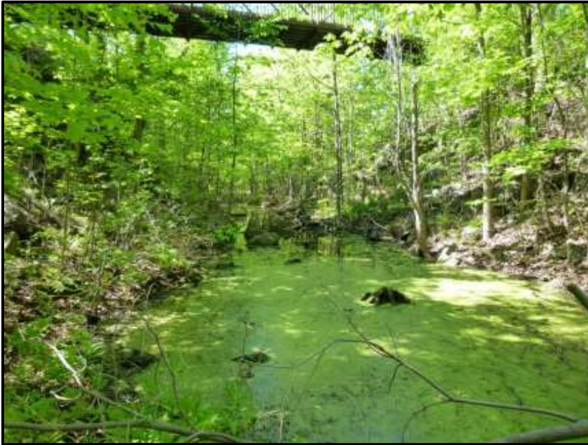
Photograph 110: Stormwater Infiltration Swale within Section #6. The Stormwater Infiltration Swale is fed by a pipe from the adjacent subdivision. The Section #6 Stormwater Infiltration Swale has no outlet, and standing water infiltrates/evaporates (May 24 th , 2018).
