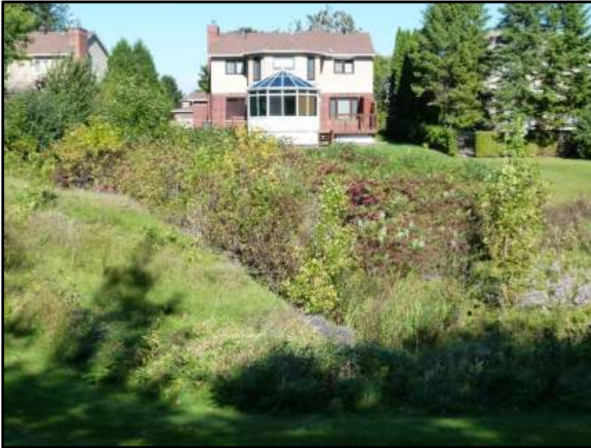
Photograph 113: Dry Stormwater Infiltration Swale within Section #3 – no surface water observed (September 17 th , 2018).
