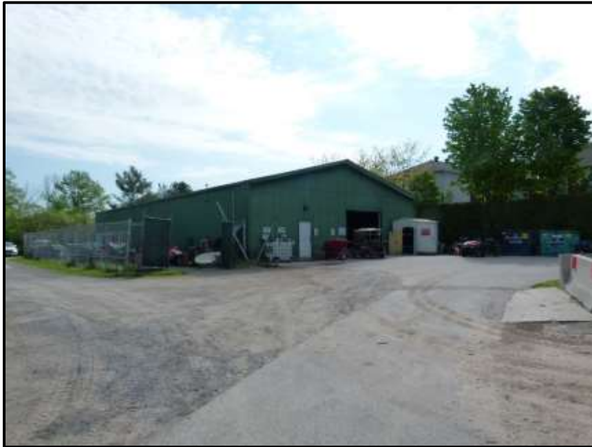
Photograph 121: Looking east at Building #1. The garage door is closed on a nightly basis (May 24 th , 2018).
