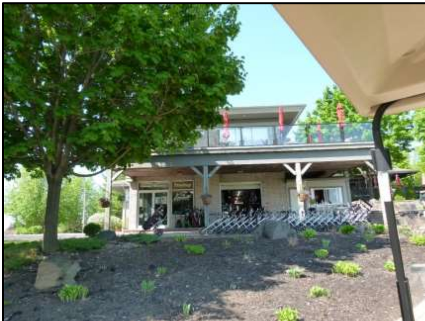
Photograph 123: Looking west at Building #3 (May 24 th , 2018).
