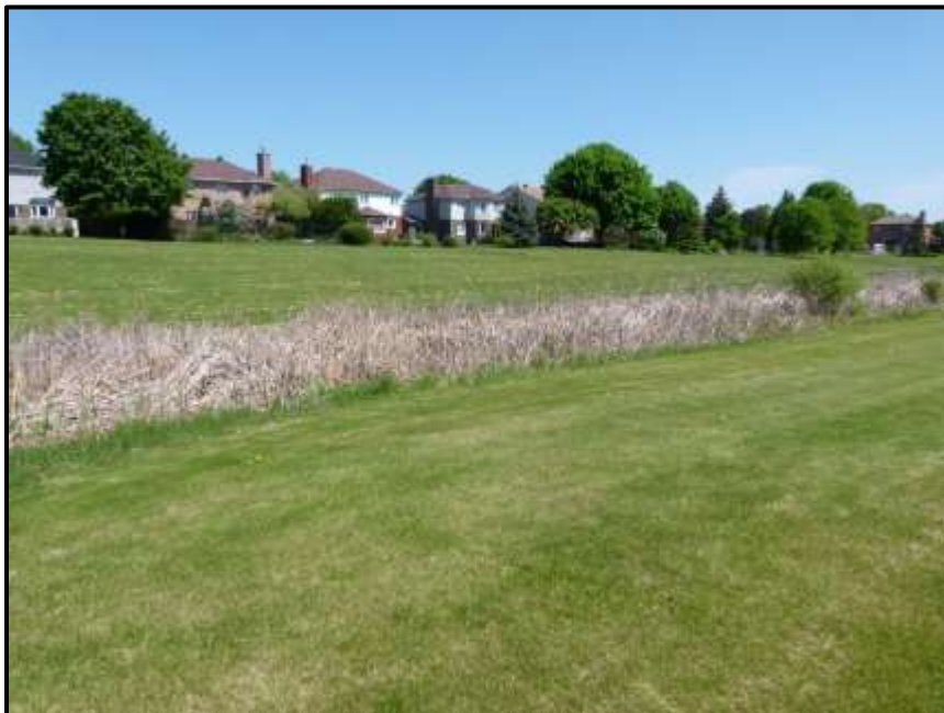
Photograph 112: Dry Stormwater Infiltration Swale within Section #3 – no surface water observed (May 24 th , 2018).
