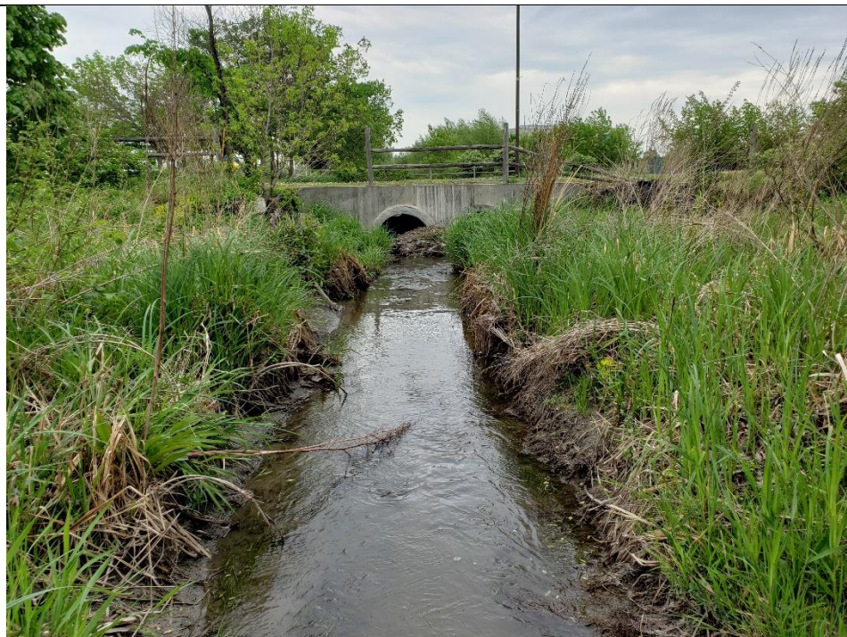
View downstream of beaver dam where the exposed silt and clay toe of bank can be observed
