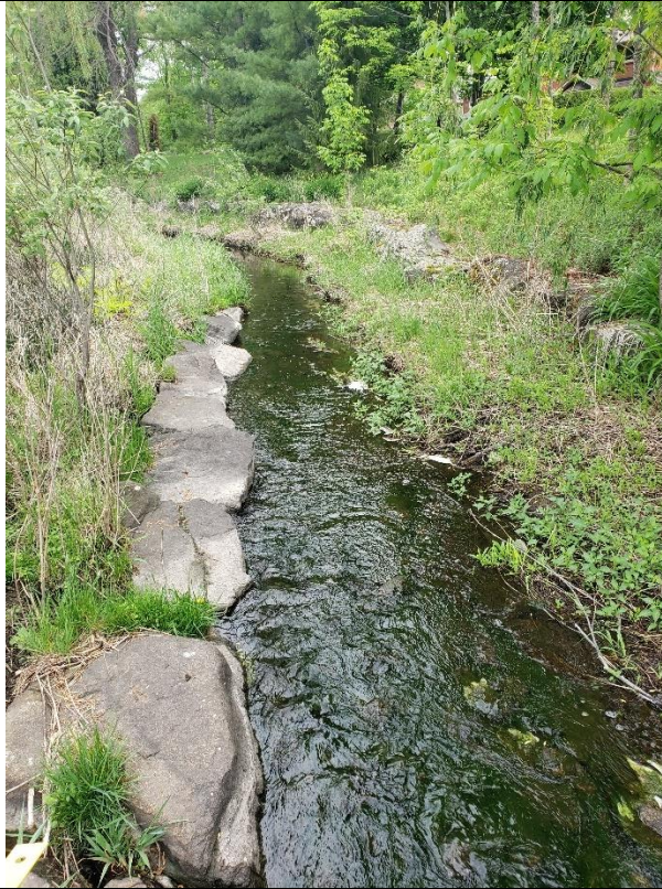
Looking downstream at the furthest upstream extent of Site KDR-4, immediately downstream of the Beaver Pond outlet. Both banks are armoured and vegetated.
