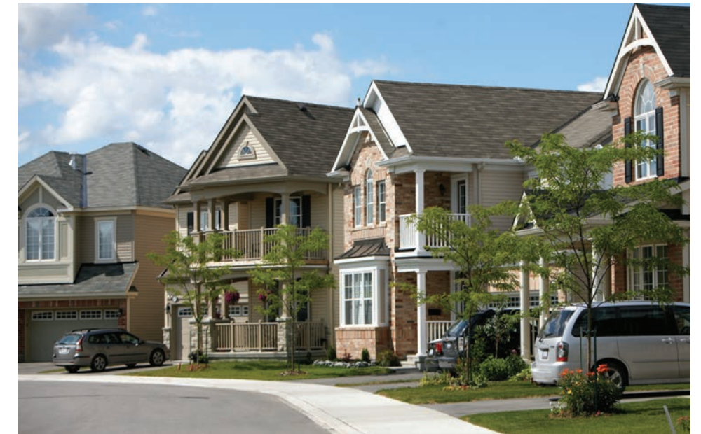
Primary Sidewalk Condition
