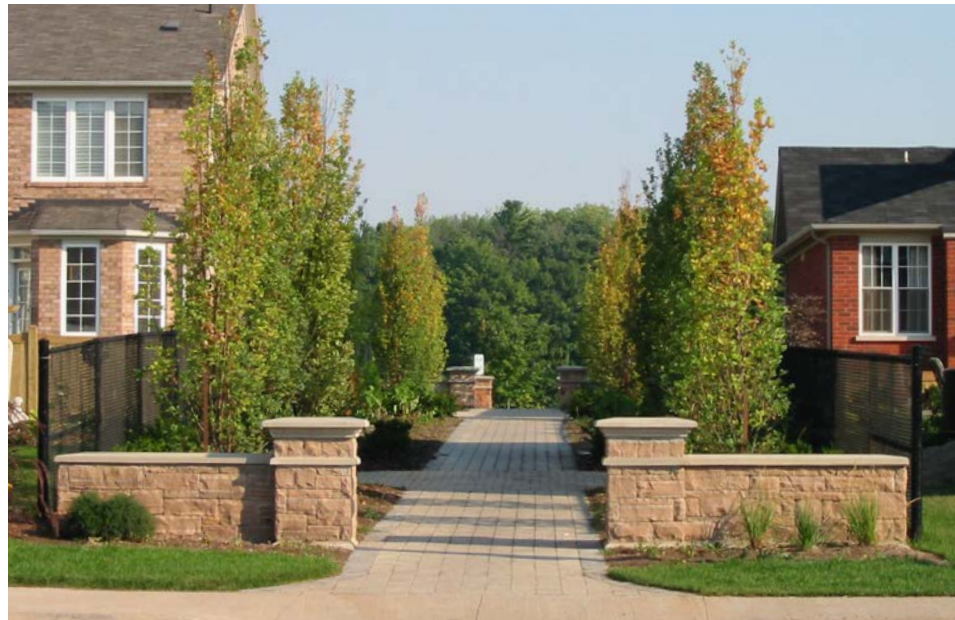
Walkway Block Condition
