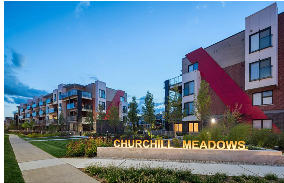
Gateway Entry Feature
