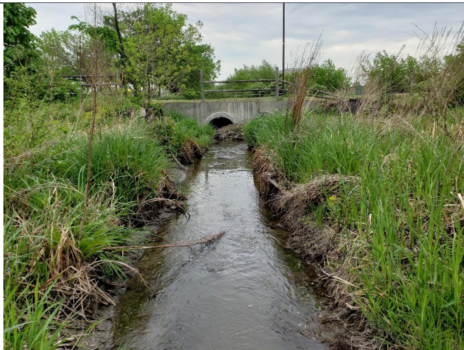
View downstream of beaver dam where the exposed silt and clay toe of bank can be observed
