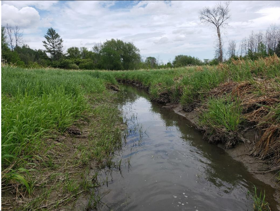
Through KDR-1, there is evidence of lateral migration. In this photograph (looking downstream), deposition of sandy silts were observed along the left bank and slumping was observed along the right bank.
