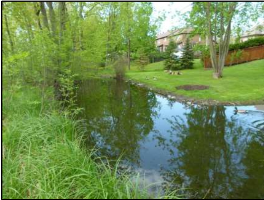
Photograph 108: Stormwater Infiltration Swale within Section #5. The Stormwater Infiltration Swale is fed by a pipe from the adjacent subdivision, and the swale outlets to the Northern Stormwater Management Pond (May 24 th , 2018).
