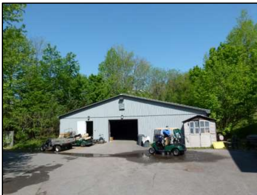
Photograph 144: Looking north at Building #2. The garage door is closed on a nightly basis. No significant exterior openings were noted (May 24 th , 2018).
