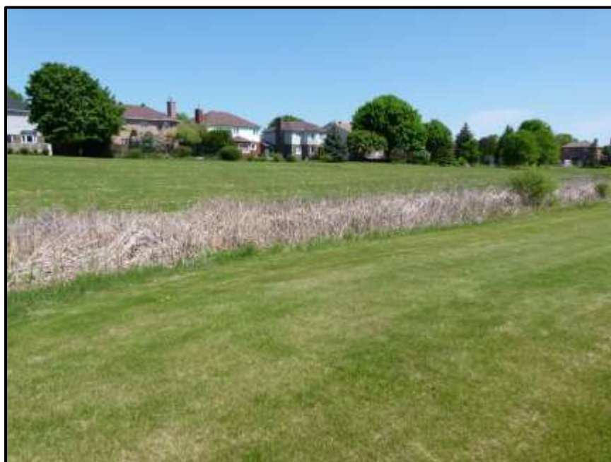
Photograph 112: Dry Stormwater Infiltration Swale within the southern part of Section #3 – no surface water observed (May 24 th , 2018).
