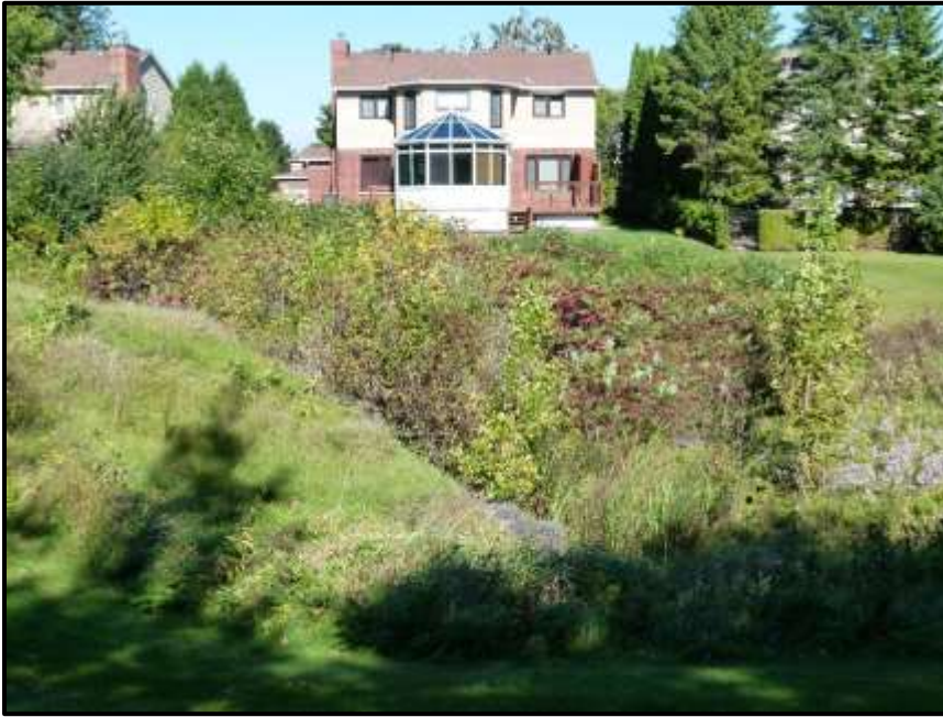
Photograph 113: Dry Stormwater Infiltration Swale within the northern part of Section #3 – no surface water observed (September 17 th , 2018).
