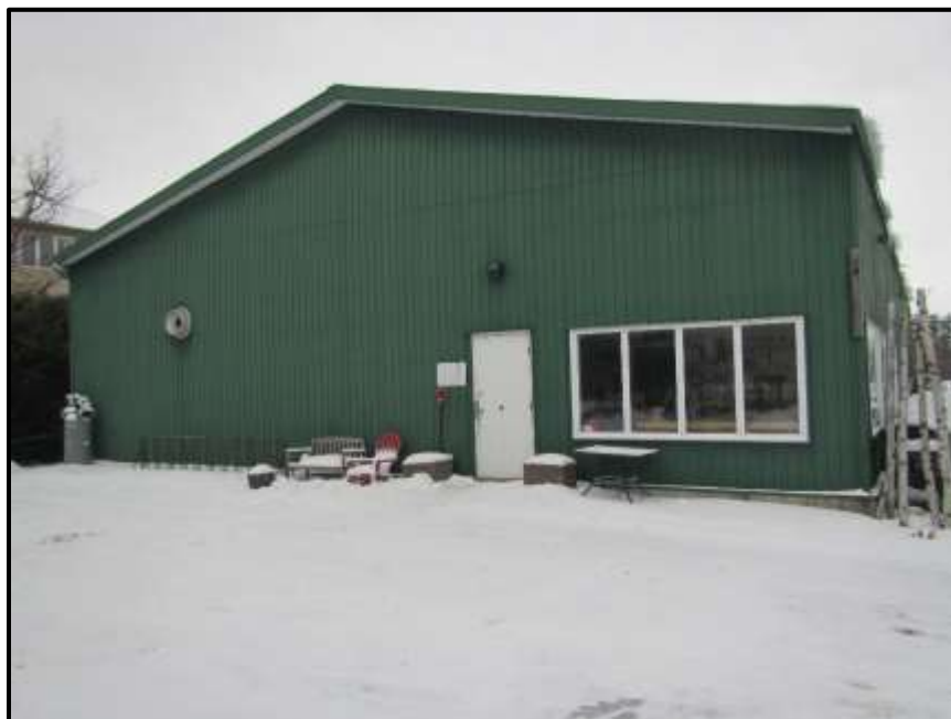
Photograph 143: Looking west at Building #1. No significant exterior openings were noted (January 10 th , 2020).
