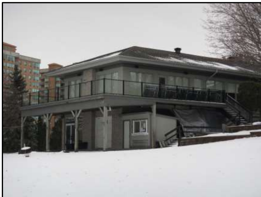
Photograph 145: Looking southwest at Building #3. No significant exterior openings were noted (January 10 th , 2020).
