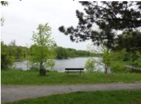
Existing Stormwater pond
