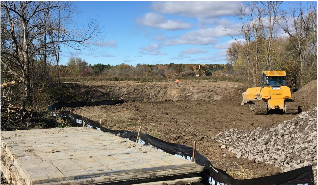
Photograph 4: View of the central portion of the subject site, looking west.
