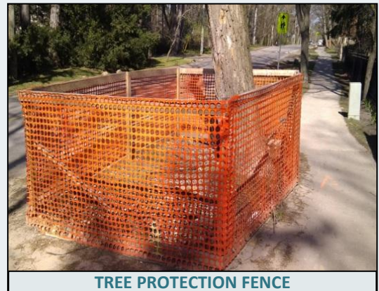
TREE PROTECTION FENCE
