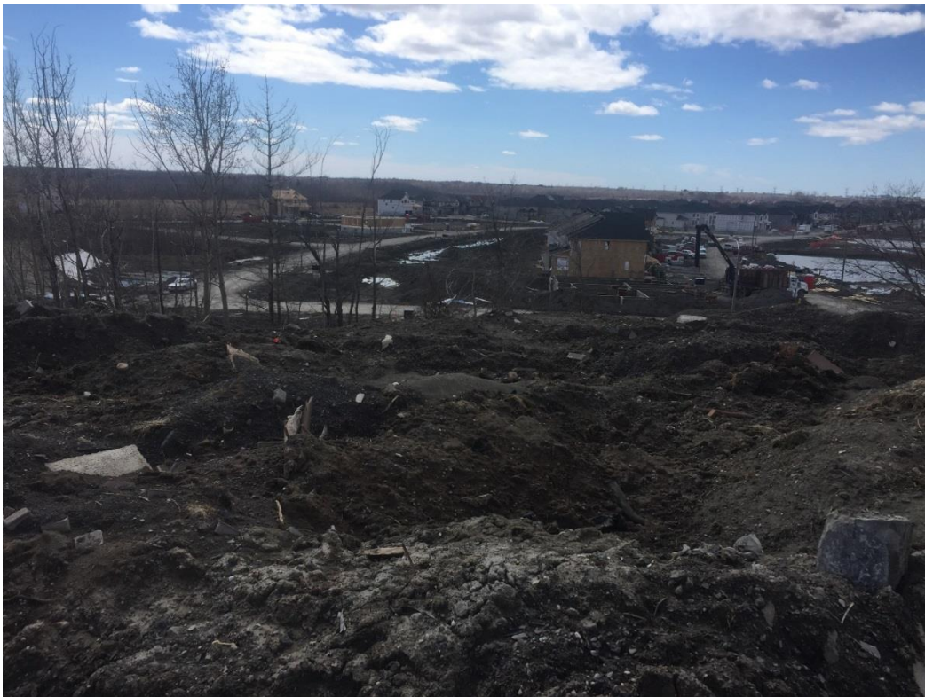
Photograph 4: Central portion of the site, facing west
