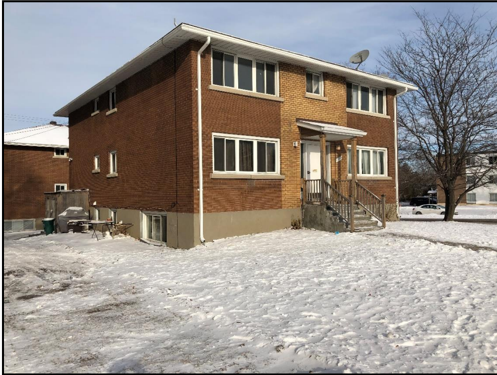
Photograph 1: View of the Phase I Property, facing north from Carling Avenue.
