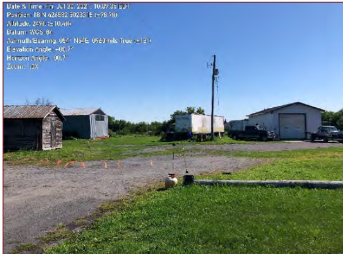
Site Photograph 11 – Previous Development On-site
