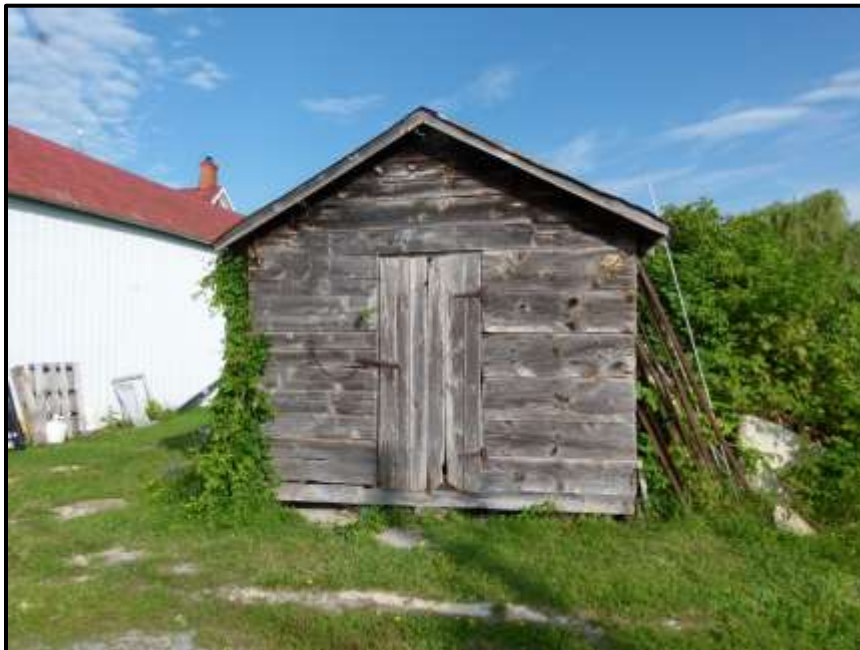
Photograph 20: Building #2 – no Barn Swallow nests were noted (August 14 th , 2017).
