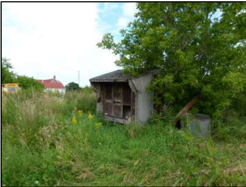
Photograph 28: Building #9 – no Barn Swallow nests were noted (August 14 th , 2017).
