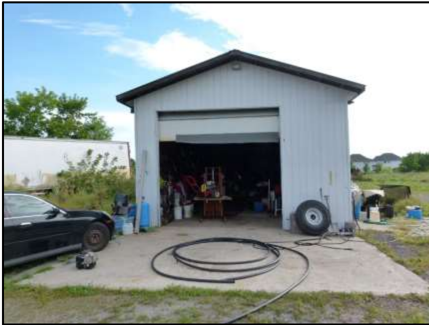
Photograph 21: Building #3 – no Barn Swallow nests were noted (August 14 th , 2017).
