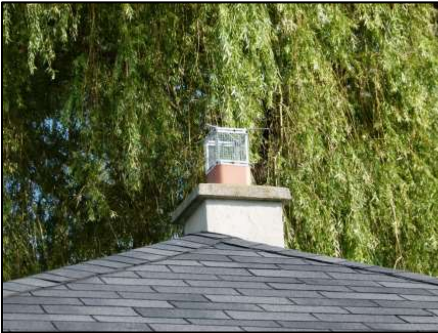
Photograph 31: 920 March Road (Building #5) chimney with metal cap (August 14 th , 2017).
