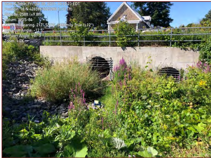
Site Photograph 9 – Inlet for Tributary 4
