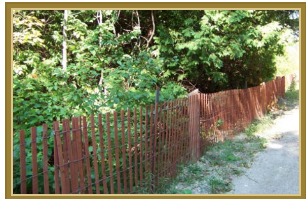
Plate 5. Example of a wood lath snow fencing used to exclude turtles (photo credit: Karine Beriault).
