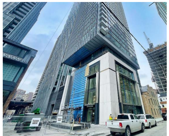
Figure 3. The building at 8 Cumberland Street in Toronto, which has a cantilever above a mid-block pedestrian connection POPS. The cantilever is located on level 6.
