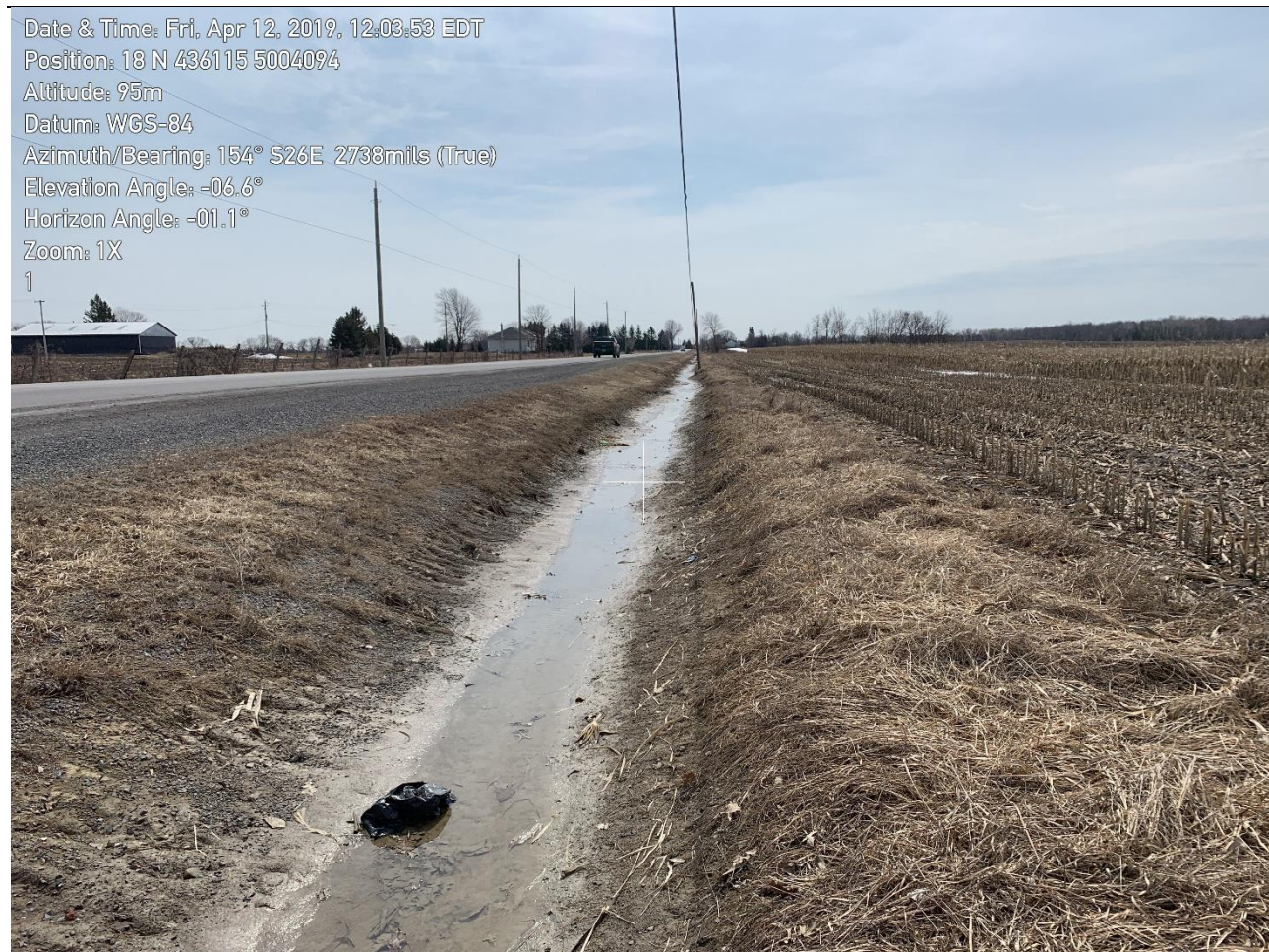
Figure 4 Photo showing the roadside ditch along Eagleson Road taken on April 12, 2019
