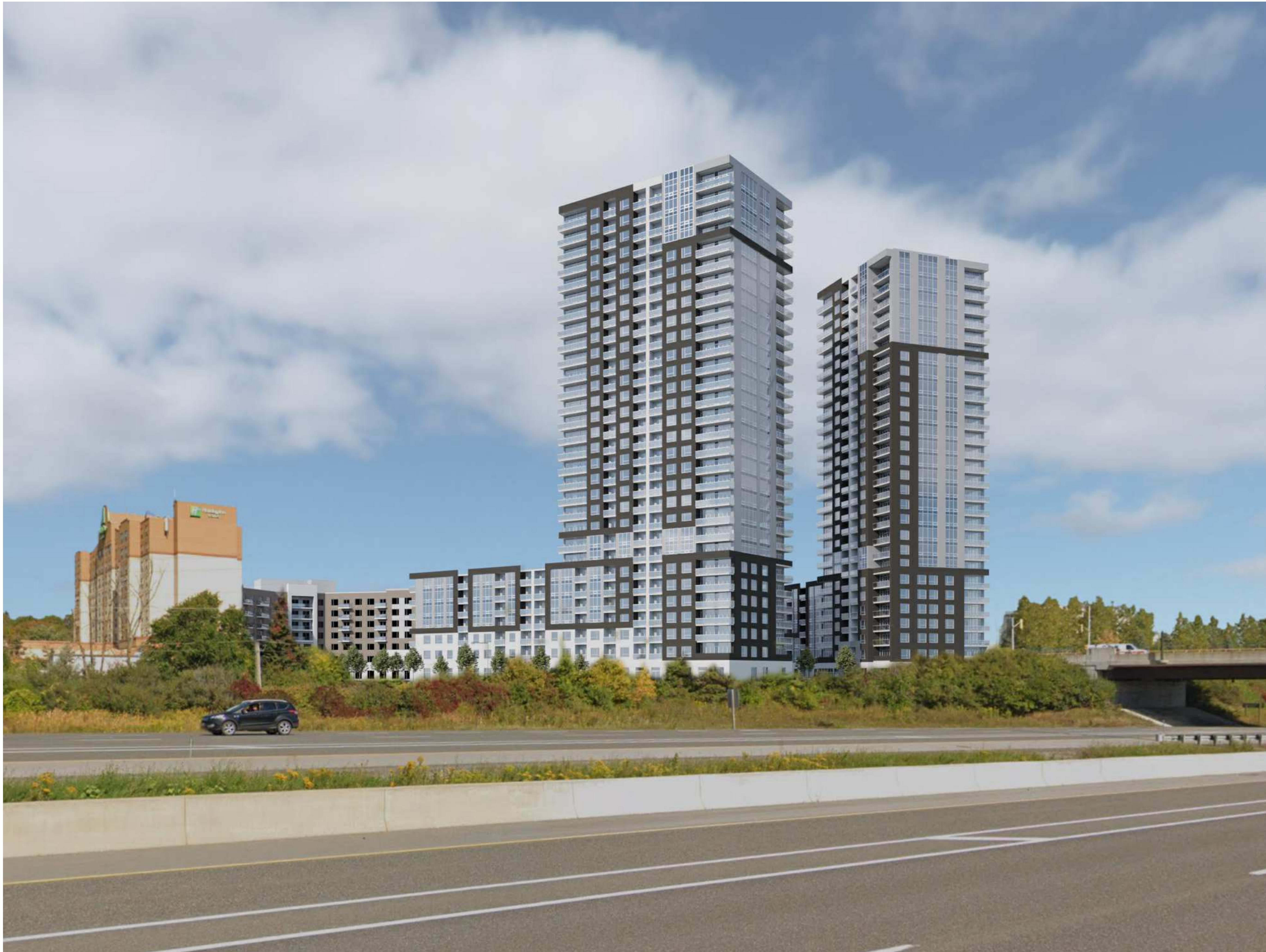
STREETSCAPE LOOKING EAST
