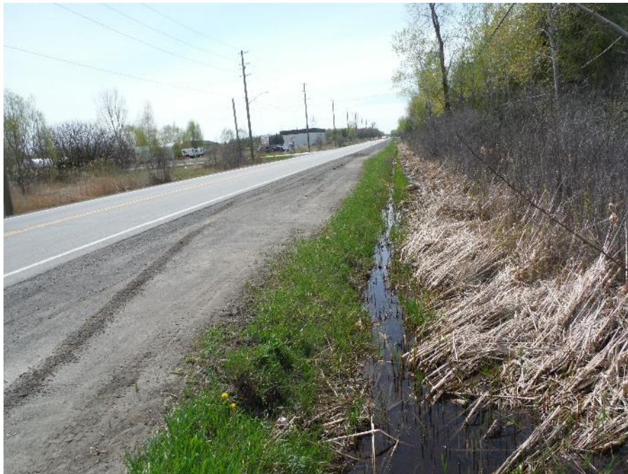
Photo 1: Roadside ditch, looking south (May 17, 2020)
