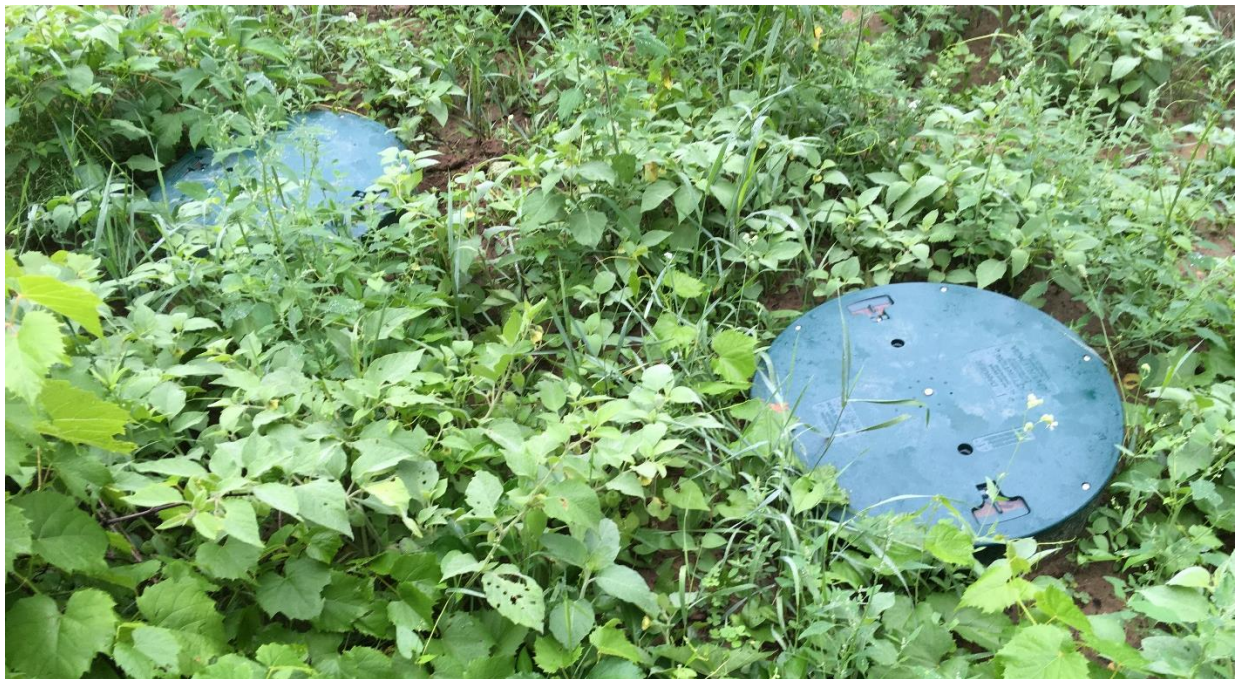
Photograph 14: View of the septic system, located on the north side of the residential dwelling.
