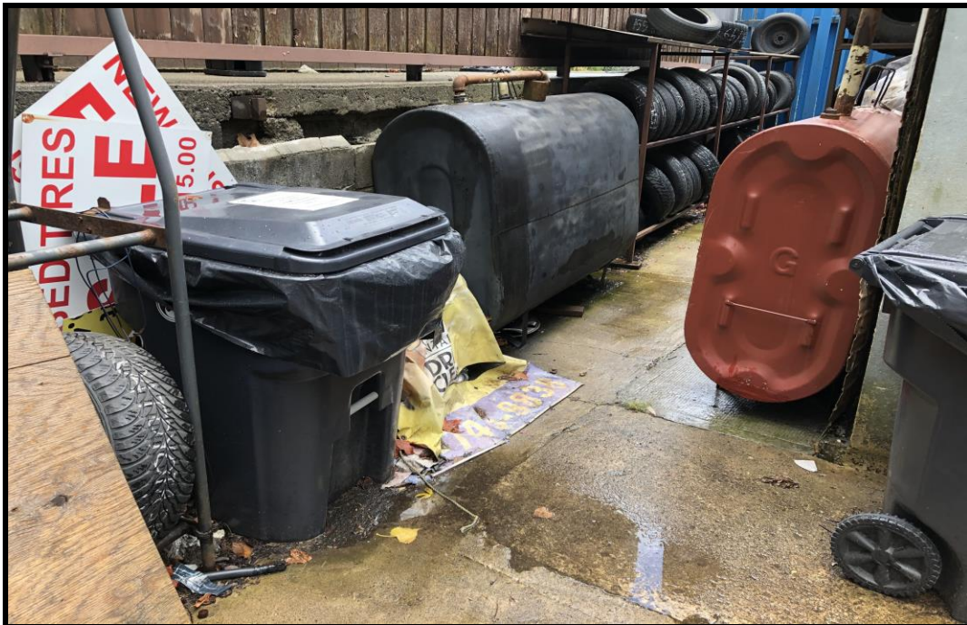
Photograph 6: View of two (2) aboveground waste oil storage tanks, located on the rear exterior of the auto service garage, facing south.
