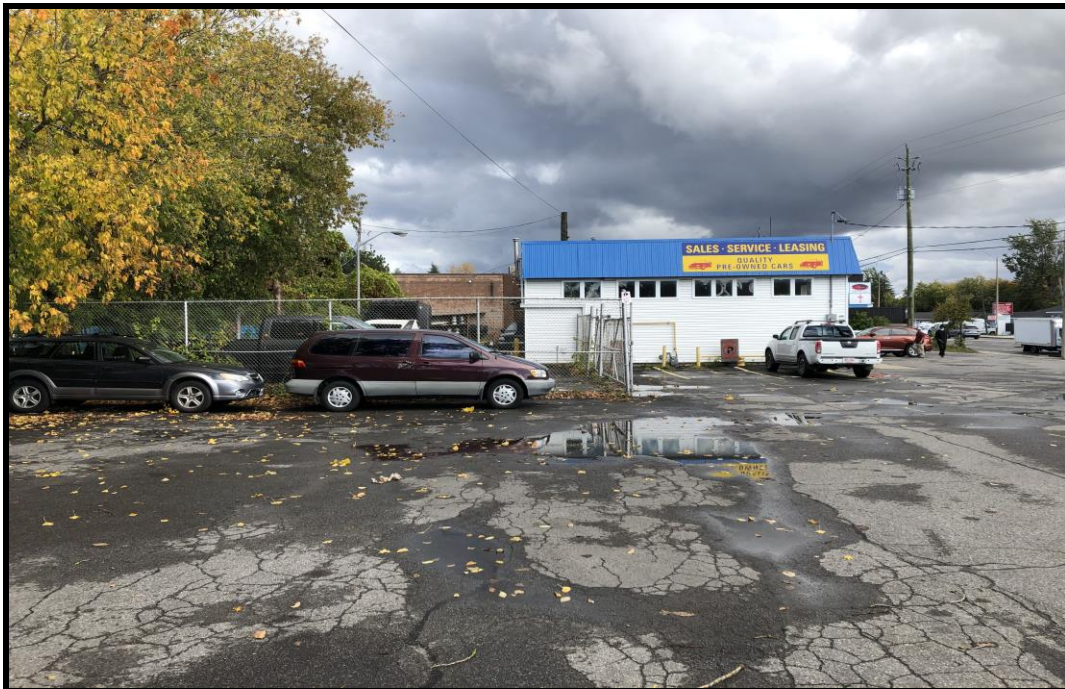
Photograph 2: View of the auto service garage located at 1649 Montreal Road, facing east from Blair Road.
