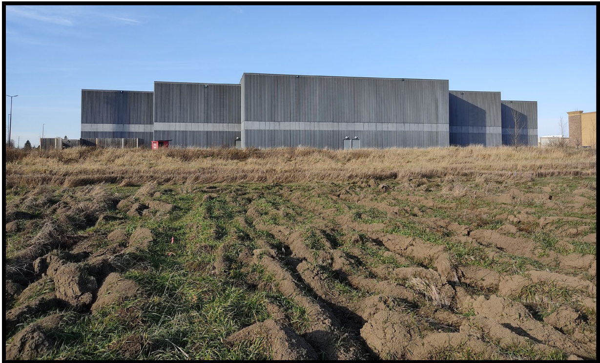
Figure 1: Overview of the Mahar site area (D07).
