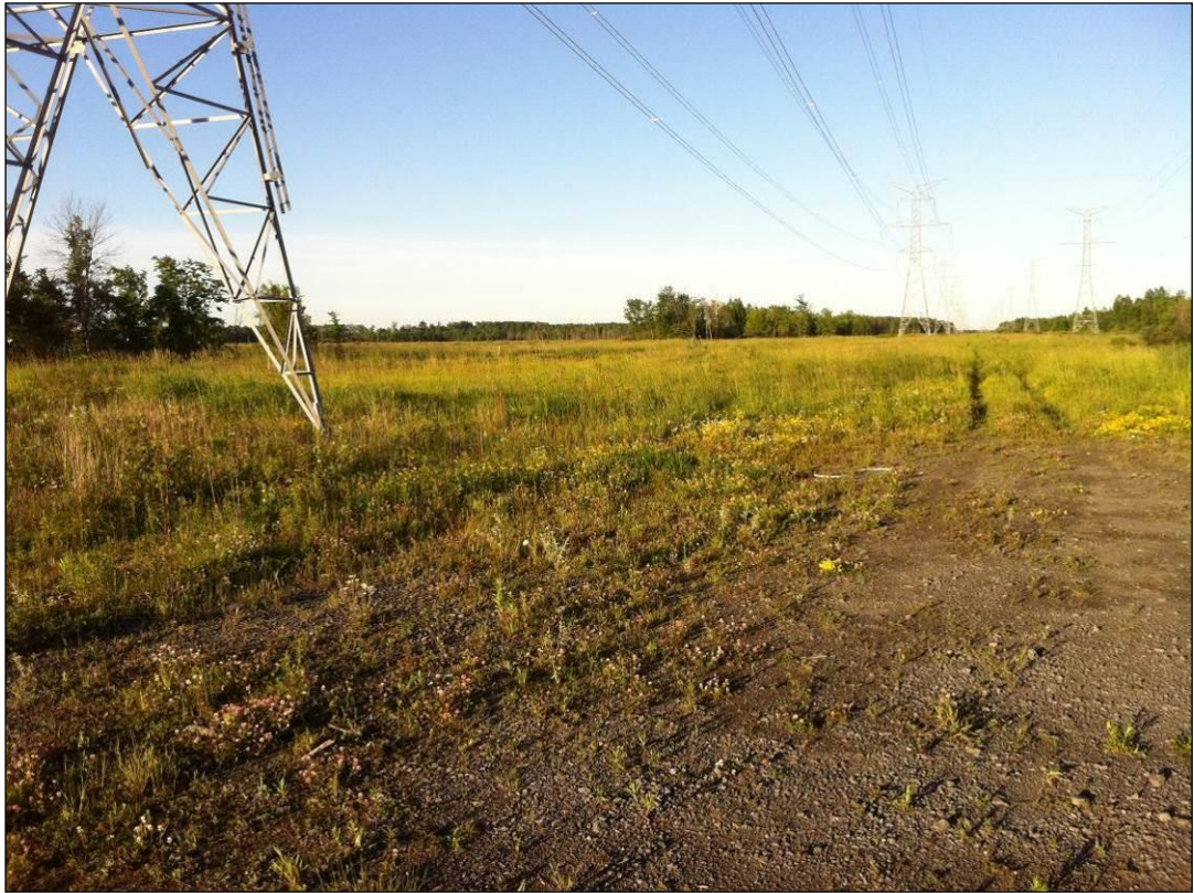
Photo 13: Hydro corridor (Photo date: May 29 th , 2014).
