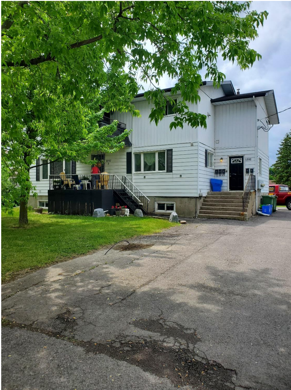
Photo 1: Facing west, the “site” consists of a two storey residential building with five (5) apartments. Northern portion of the site is asphalt covered and serves as a parking area for the residents.
