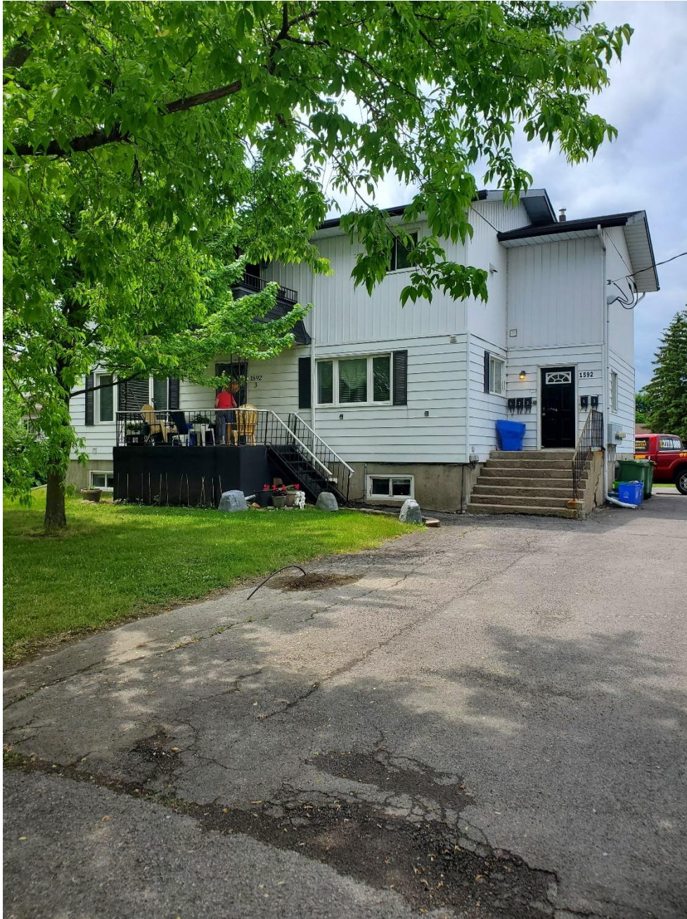
Photo 1: Facing west, the “site” consists of a two storey residential building with five (5) apartments. Northern portion of the site is asphalt covered and serves as a parking area for the residents.
