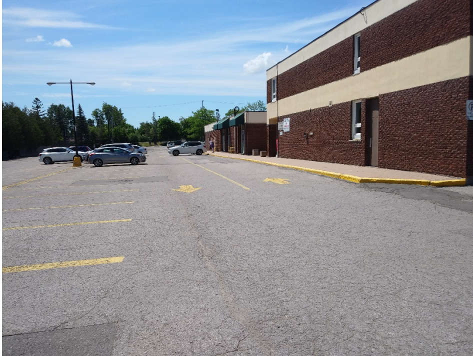
Photograph 5: View of the east side of the Phase One Property looking south. View shows the east sides of the north and south commercial buildings.
