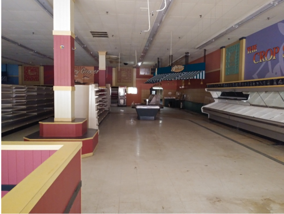
Photograph 11: View of interior of the former grocery store in the northwest portion of the north commercial plaza building.
