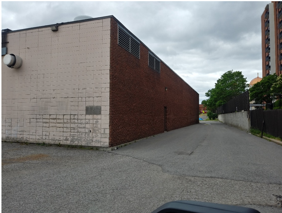
Photograph 4: View of the west side of the Phase One Property looking south. View shows the west side of the north commercial building.
