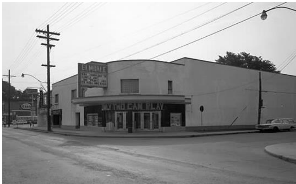
19 Elmdale Theatre, corner of Hamilton Ave N and Wellington St W, 1962. City of Ottawa Archives, CA24804.
