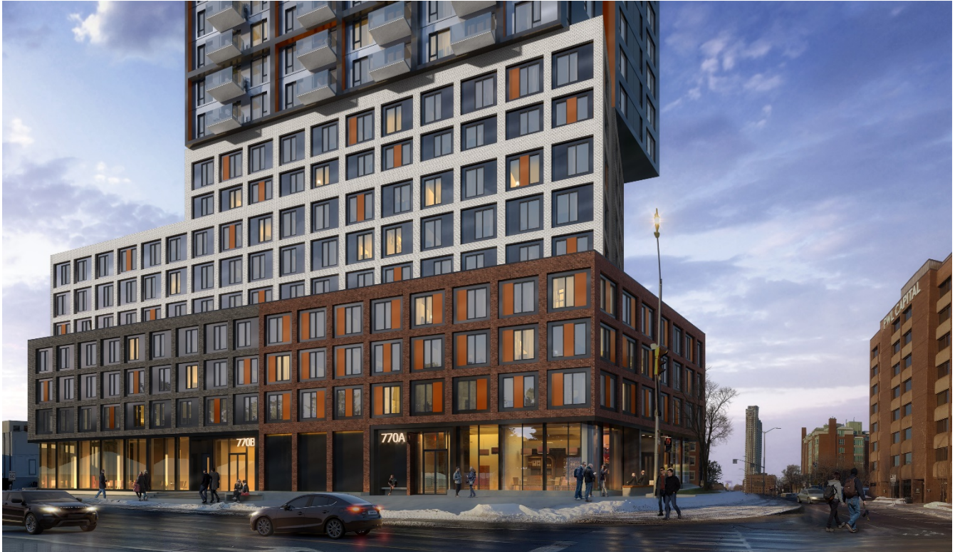
Figure 7: View of Proposed Development, Looking West from Bronson Avenue at Glebe Avenue
