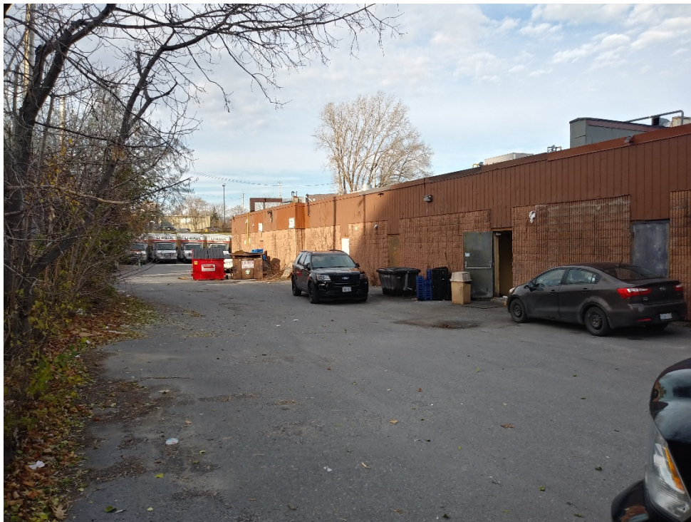
Photograph 2: View of west portion of the Phase One Property, looking north.
